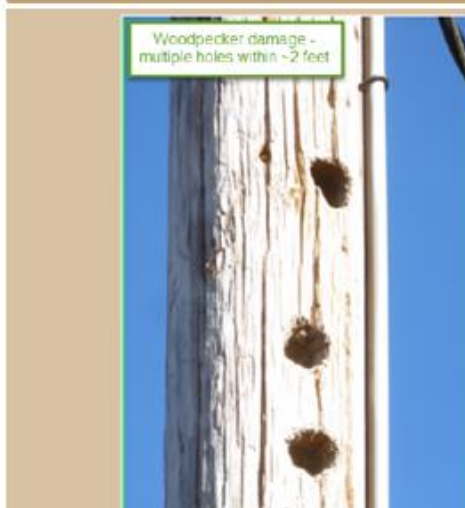
Woodpecker damage - large cavity
