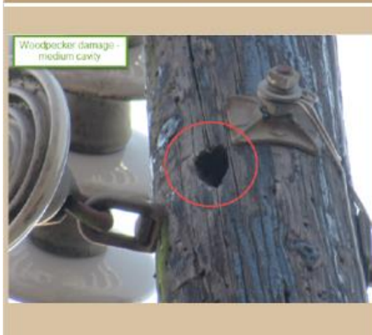
Woodpecker damage - medium cavity
